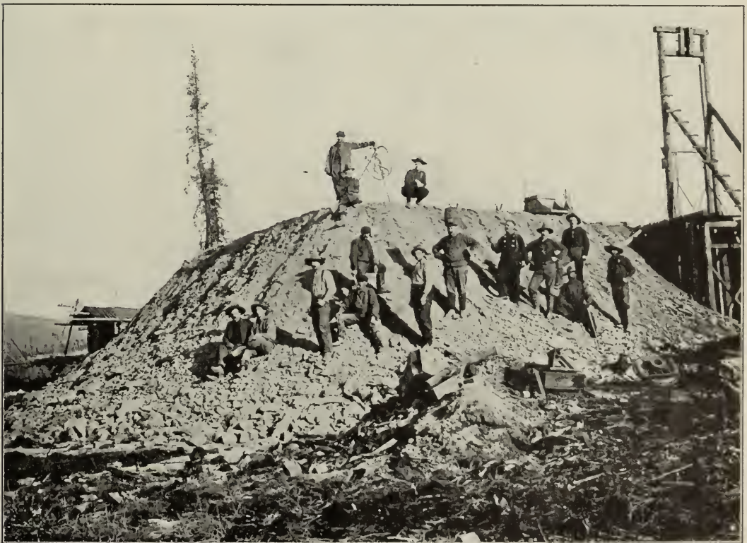
NO. 16 ELDORADO, SHOWING DUMPS OF GRAVEL THAWED BY STEAM AND HOISTED. THE CLAIM IS BEING WORKED BY A DREDGE.
